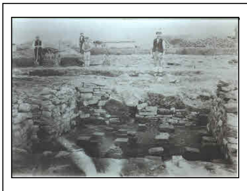
Andrew and Lees excavation team. 1908
