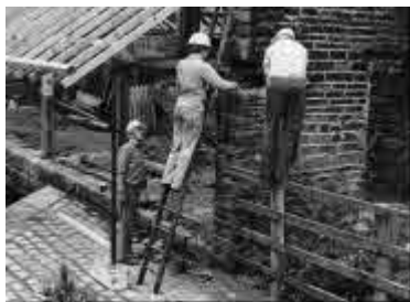
The Warehouse During Restoration
