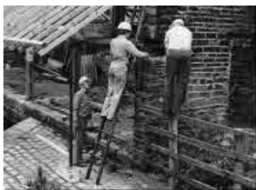
The Warehouse During Restoration
