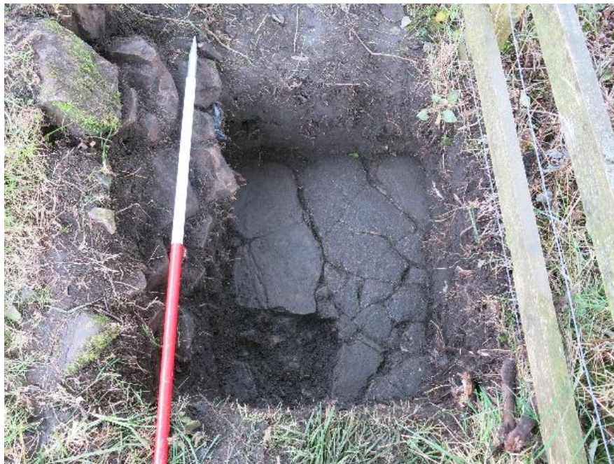
TP19 excavated in 2021, showing the smooth tightly jointed gritstone surface.
