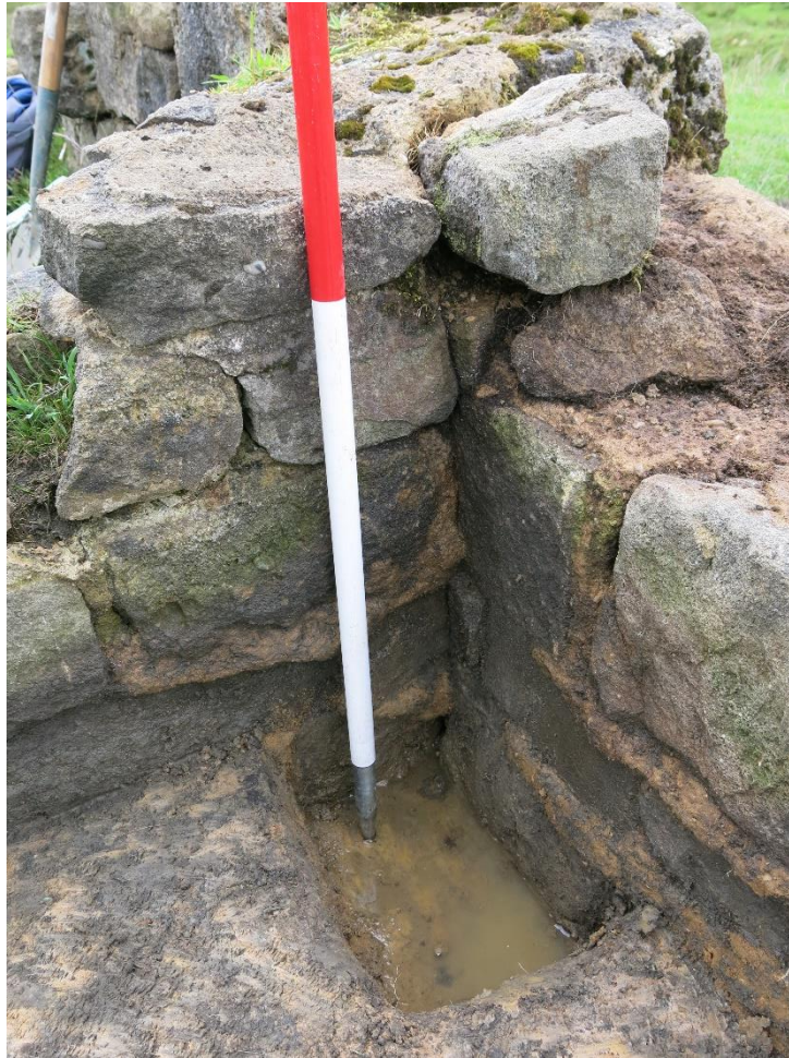
Detailed view of north west corner of corridor in TP7 showing butt joint and five courses of stonework
