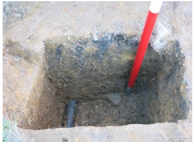
TP 1 looking north with the cut of the pipe trench clearly visible (left) and a section dug through the trench to reveal the plastic pipe (right)
