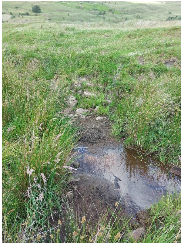
Prior to clearance work, the stepped stonework can be seen on the far side of the clough. Looking west.
