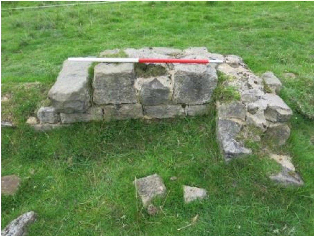
The north-west corner of the ruin, showing the nature of stone coursing and thickness of the walls. The gritstone blocks are crudely dressed and in places larger stones extend the full width of the wall, as in the example top right of the photo.
